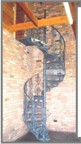
An overall view of a staircase consisting of 16 steps and custom made top landing.
